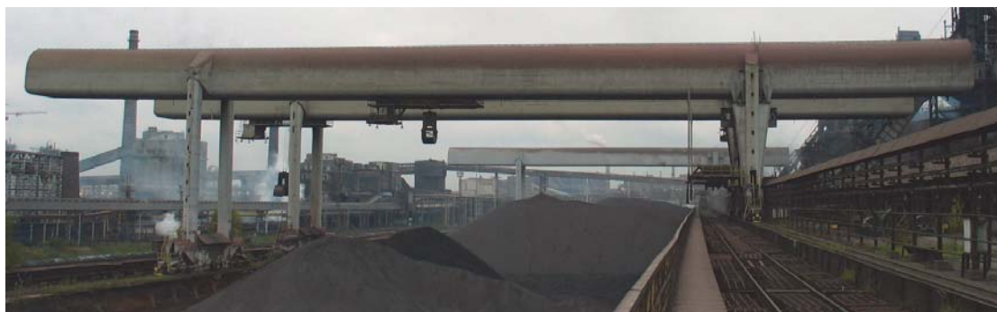
Fig. 1. Gantry cranes of a coating structure
