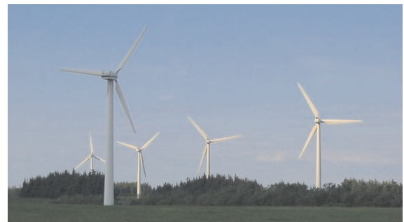
Fig. 15. General view of wind power plant (www.wikipedia.pl)
