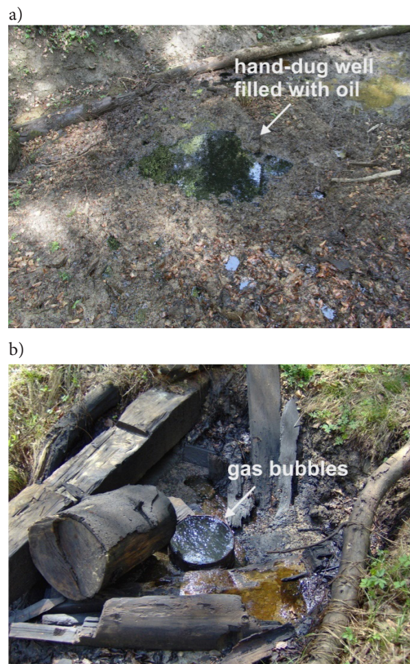
Fig. 2. An example of an old hand-dug set near Polana Ostre village: a) visible outline of the walls of the old hand-dug filled with oil; b) open outlet of the borehole with visible bubbles of methane [19 – modified]
