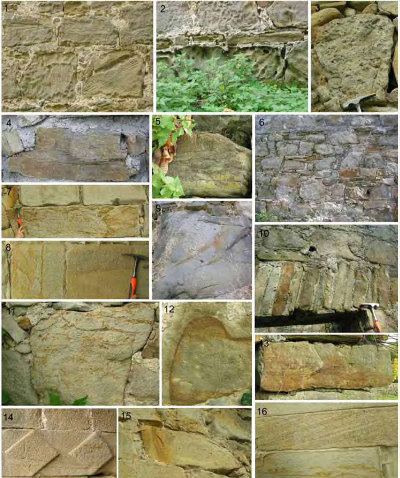
sandstone (g) with convolute lamination; 6 – part of wall built of coarse-grained sandstones with parallel lamination in places (i) and fine-grained, tabular sandstones with parallel and cross lamination (i, g); 7 – water-escape sedimentary structures within coarse-grained sandstone (i); 8 – sharp boudary between coarse-grained and medium-grained sandstone (i); 9 – flute-casts (good indicators of paleo-currents directions) on a bottom surface of sandstone layer (g); 10 – “briquettes” from darker, brownish, fine-grained sandstones (g) and lighter, tabular, coarse-grained sandstones (i) in stone door-frame; 11 – water-escape structures within coarse-grained sandstone (i); 12 – coarse-grained sandstone with single grains of glauconite (?g); 13 – coarse-grained massive sandstone passing to fine-grained up top of layer (g) – part of layer in overturn position (top turned down and bottom turn up); 14 – decorative ornamentation of stone door-frame made of coarse-grained sandstone with cross-lamination (i); 15 – coarse-grained sandstone (i); 16 – cross-laminated and massive coarse-grained sandstone (i).
