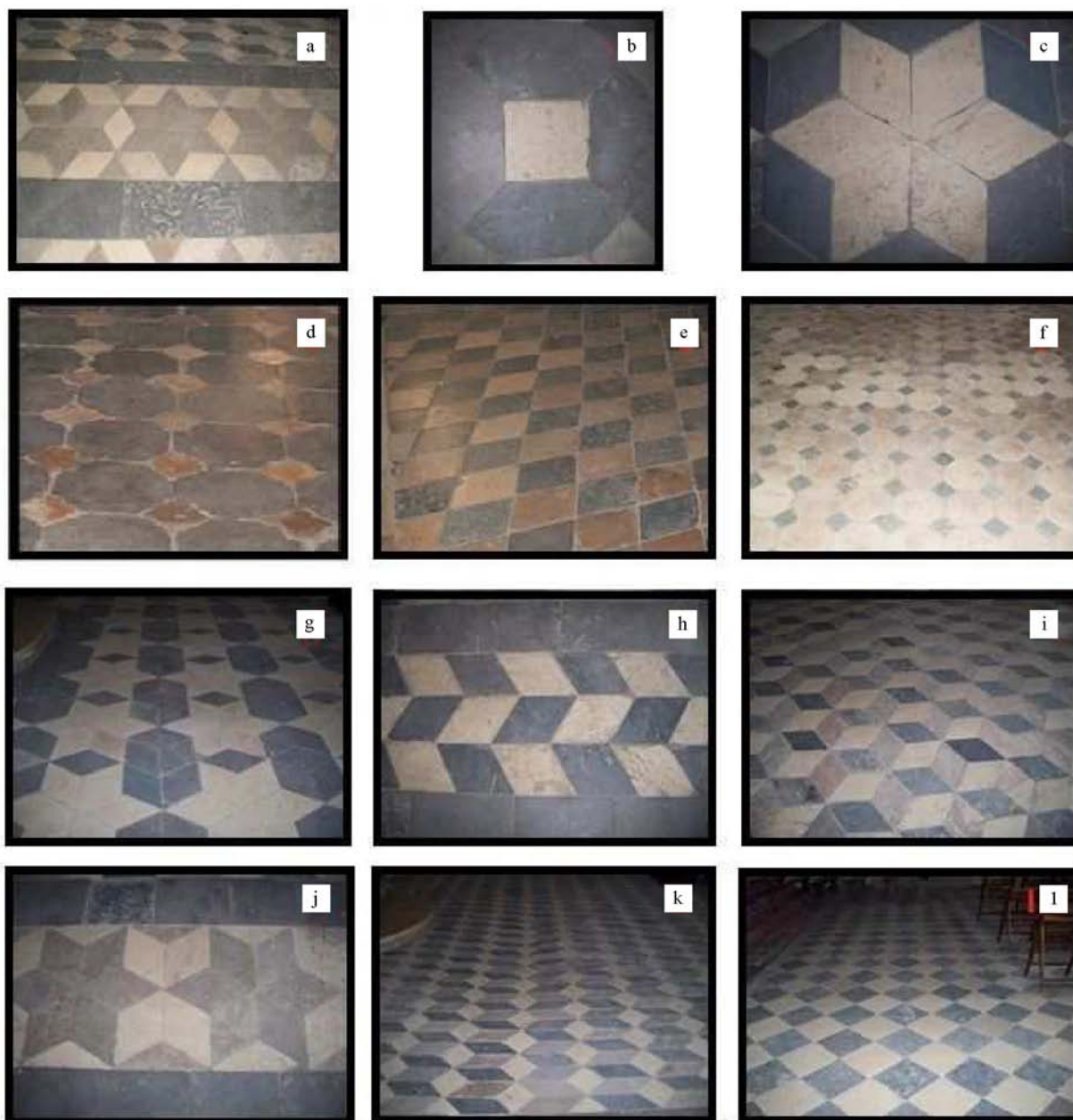
Fig. 8. The stone material used in the floor tile patterns, phot. M. Florczyk: a. A row of stone tiles made of the black Devonian limestone separating floor parts of various tile patterns; b. The main nave – the black Dębnik Limestone and the creamy Jurassic limestone; c. The passage between the main nave and the transept – the creamy Jurassic limestone; d. The transept – the black Dębnik Limestone and the brown Bolechowice Limestone; e. The transept part adjacent to the chancel – the black Dębnik Limestone and the brown Bolechowice Limestone; f. The narthex of the left aisle – the creamy Jurassic limestone and the black Dębnik Limestone; g. The chapel of St. Sebastian – the creamy Jurassic limestone and the black Dębnik Limestone; h. The passage into the chapel of St. Catherine of Alexandria – the black Dębnik Limestone and the creamy Jurassic limestone; i. The chapel of St. Catherine of Alexandria – the black Dębnik Limestone, the pink limestones from Chęciny and the creamy Jurassic limestone; j. The passage into the chapel of St. Peter in Vinculi – the brown Bolechowice Limestone and the creamy Jurassic limestone; k. The chapel of St. Peter in Vinculi – the black Dębnik Limestone, the brown Bolechowice Limestone and the creamy Jurassic limestone; l. The chapel of the Holy Cross – the creamy Jurassic limestones and the black Dębnik Limestone
