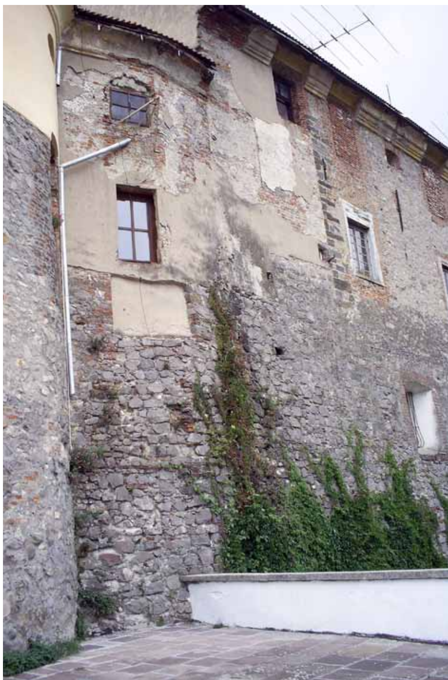
Fig. 8. Walls of the Palanok Castle built of andesitic rocks. (Lanskyi, 2009) • Mury zamku Palanok zbudowane z andezytów
