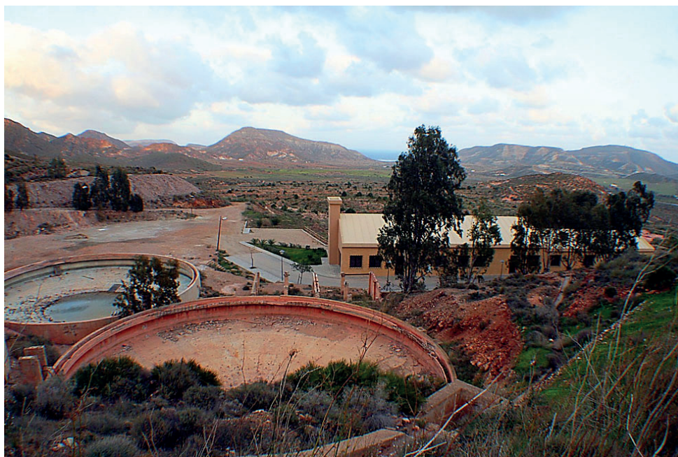
Fig. 7. The remains of the Rodalquilar gold mine: circular in shape cleaning tanks for mixture of minerals and cyanide; interpretation center to the right (photo M.W. Lorenc)
