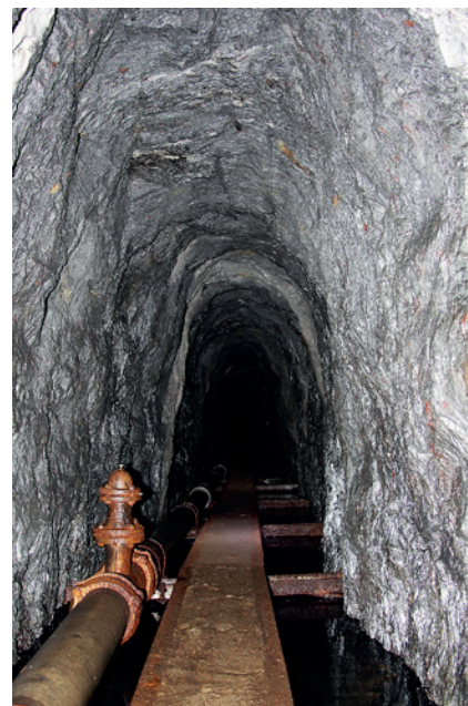
Fig. 33. Terezie water gallery at Smolnik, photo P. Hronček
