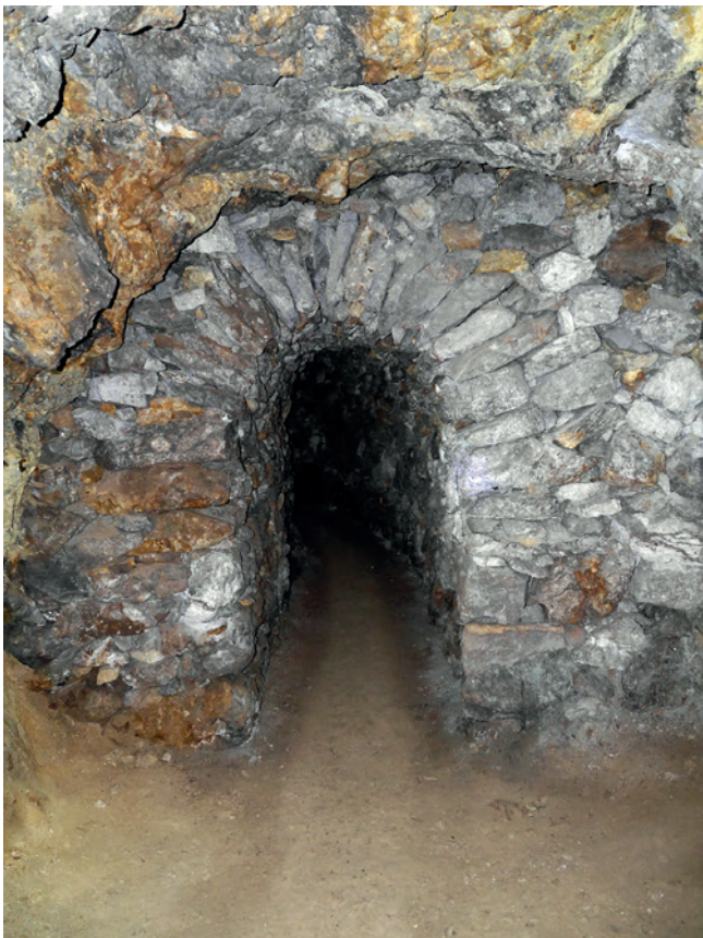
Fig. 21. Underground mining walled mine galleries on a tourist route in Starovšechsvätých mine at Hodruša Hámre (Central Slovakia), photo P. Hronček
