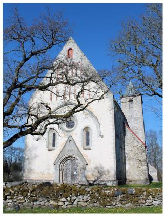
Fig. 9. Valjala Church with visible stone wall made of granite erratic boulders, photo J. Łach
