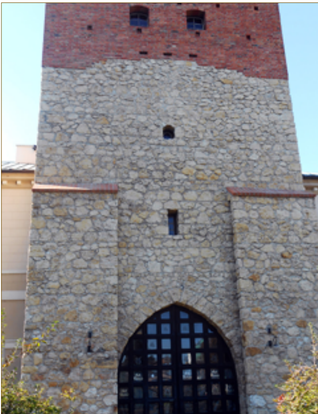
Fig. 3. General view of the Cracow’s Gate – cut stone of the Middle and Upper Jurassic limestone, photo A. Śpiewak
