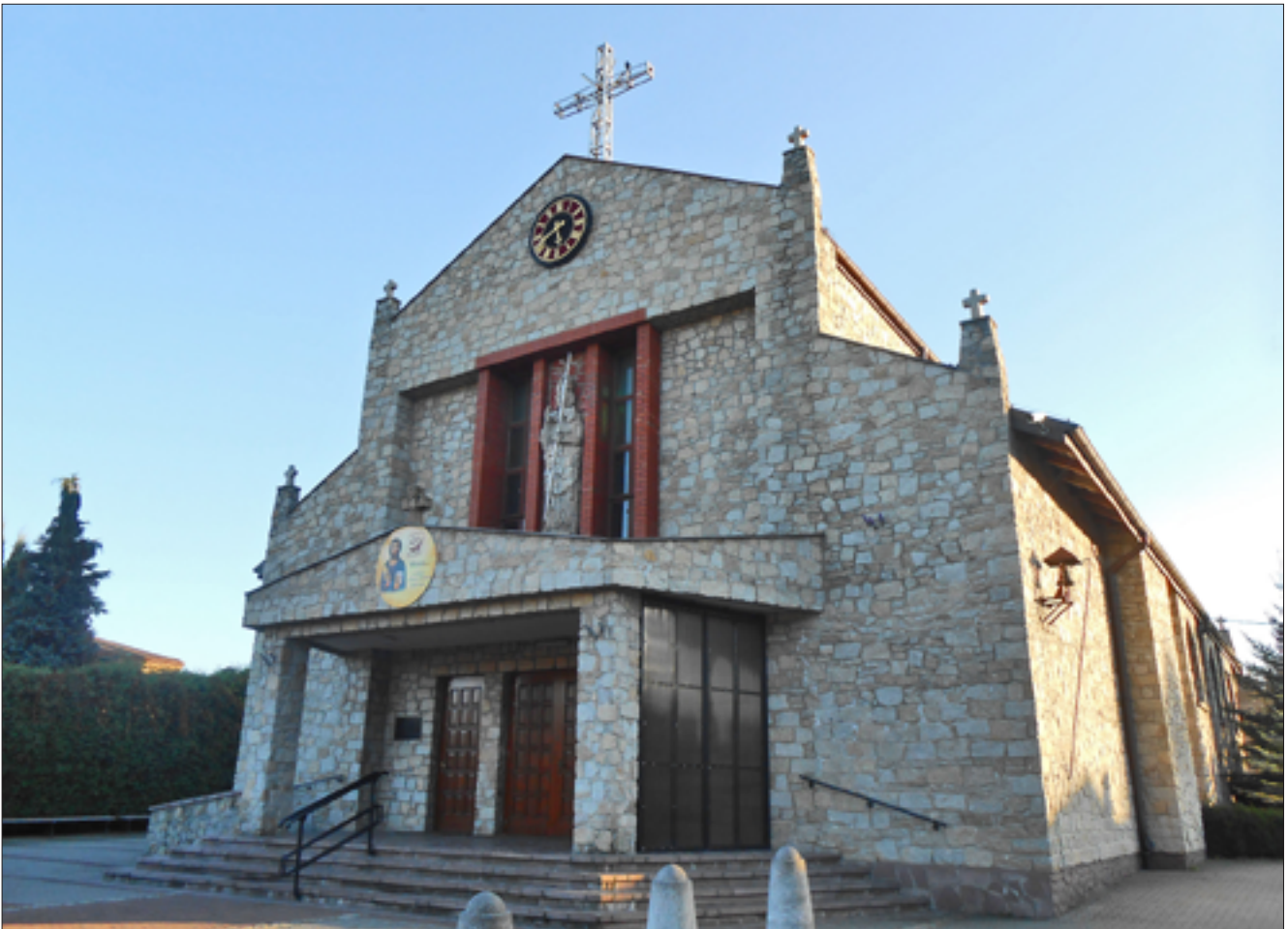
Fig. 7. The St. Stanislaus the Bishop and Martyr church, covered by Strzegom granite – general view, photo A. Śpiewak
