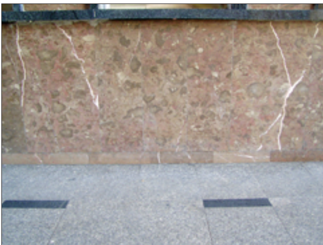
Fig. 11. The former bus station „PKS Wieluń” – vertical facing slabs of Bolechowice limestone – part of the wall and floor in the building, photo A. Śpiewak
