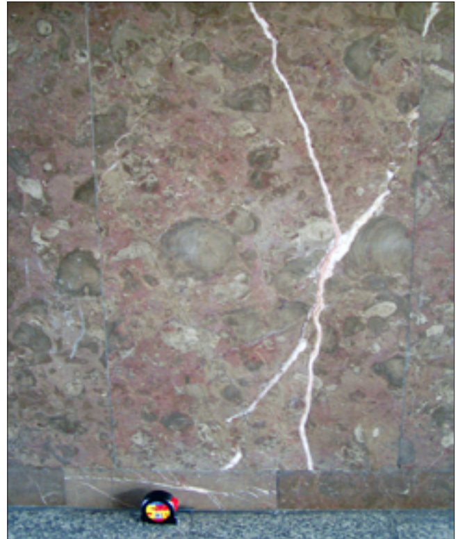
Fig. 12. A stromatoporoid structure with white and pink veins of calcite, in the slab across made of Bolechowice limestone, photo A. Śpiewak
