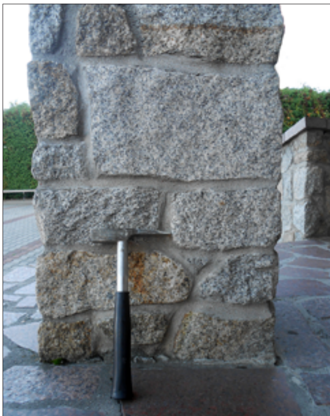
Fig. 8. The front pillar of the St. Stanislaus the Bishop and Martyr church made of Strzegom granite, with a riven surface, photo A. Śpiewak
