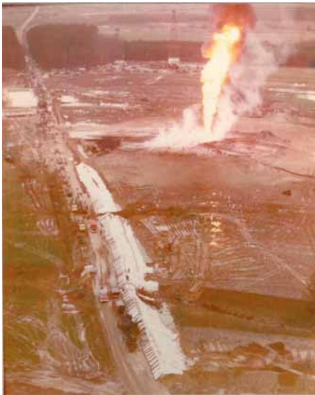
Fig. 4. General view Karlino December 1980 (source: archive of PGNIG SA in Zielona Góra)
