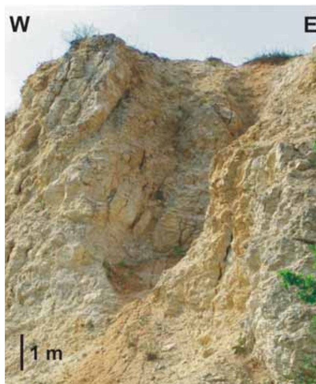
Fig. 9. Erosion-dissected karst funnel in the northern quarry wall, phot. S. Kamieniarz
