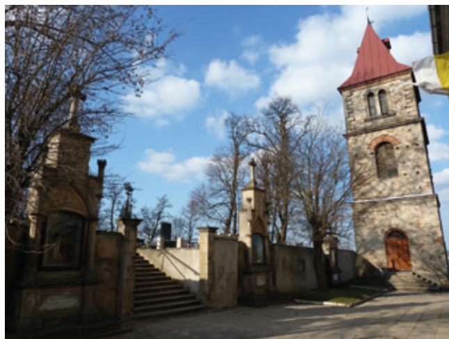
Fig. 4. Sandstone walls with gates and the Stations of the Cross around the St Władysław church, photo E. Gałka
