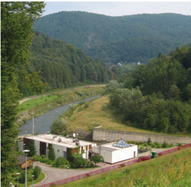
Fig. 6. Hydroelectric power station and the Ropa river valley (Gorlice Pieniny) – view from the dam crest, photo A. Waśkowska
